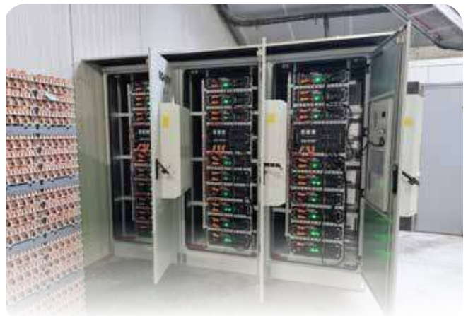
AQ-LITH® EnergyRack 138 kWh
